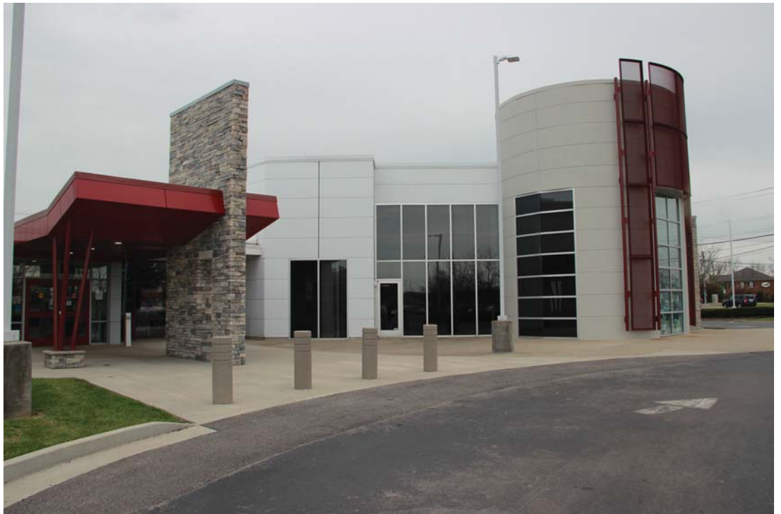
LPL's transformation of a former car dealership into the new Eastside Library is an example of a Level 3 project.
